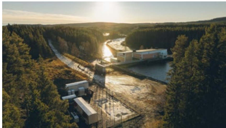
A new battery plant at the Båtfors hydropower plant provides capacity and peak load balancing in the electrical grid
