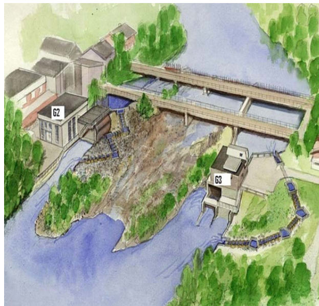
Figure 2.1.: Sketch of Power Plant. Subject of the examination are two turbines in the building on the right and the fish way next to it. In the left part of the building, the «Streamdiver» is located, in the right part «G3».
